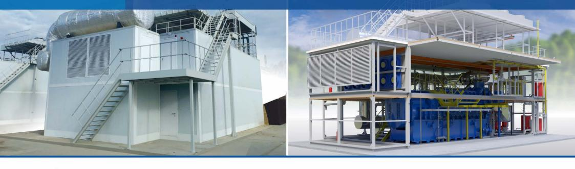
MKC® Group of Companies offers services in turnkey construction of both stationary (in a building) and modular (container) mini CHP-plants. The choice of construction technology depends on technical specifications requirements.
