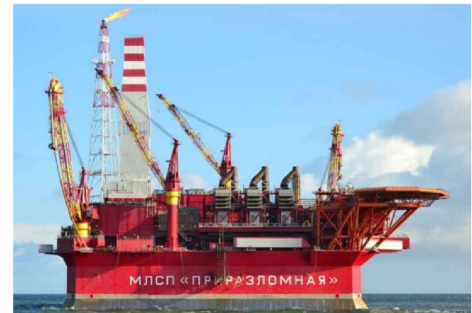
Combined flare HP/LP and gas exhaust with high content of hydrogen sulfide.
